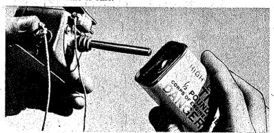
5. Insert cap in charge or, if detonating cord is used, tape one end to cap and run other end to charge.
