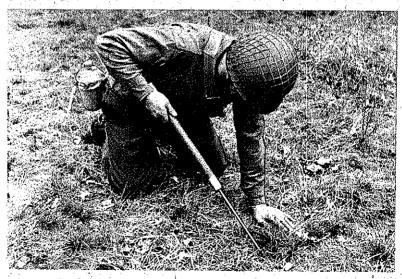
Figure 43.12c. Probing with lower half of probe M1.
