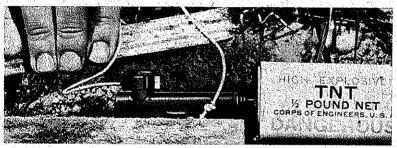
8. Remove safety pin. If pin does not come out easily, striker head probably has fallen and is pressing against it. Unscrew base and check mechanism. If defective, discard fuze and use another.
