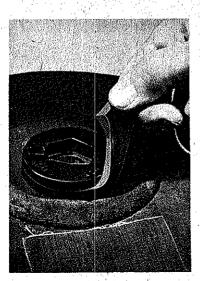
3. Place mine in hole with its surface not more than I inch below original ground surface. Remove safety ring.
