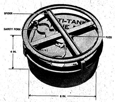
The principal difference between the two models is that in the mine M1 the booster is an integral part of the fuze; in the mine M1A1 the booster is a separate part.
