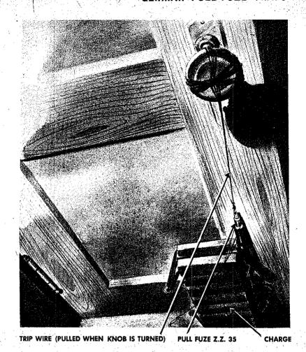
German fuzes Z. Z. 35, Z. U. Z. 35, and the various friction fuzes, are commonly used in booby traps. The above illustration of a booby-trapped door is a simple example. The charge employed usually consists of two to eight slabs of Tolite, two to eight cylindrical cartridges, an "S" mine, Tellermine, or one or more grenades, To discover these traps and disarm them—
